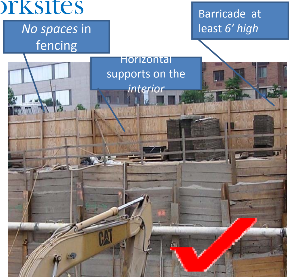
Photo from trench, looking out.
